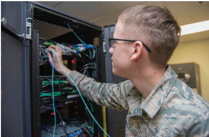
An Air Force cyber transport technician connects fiber optic cables to switches at the network control center on Holloman Air Force Base, N.M.
